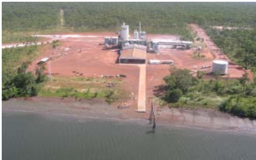
Plate 1 Port facility and kaolin processing plant at Skardon River, May 2002
