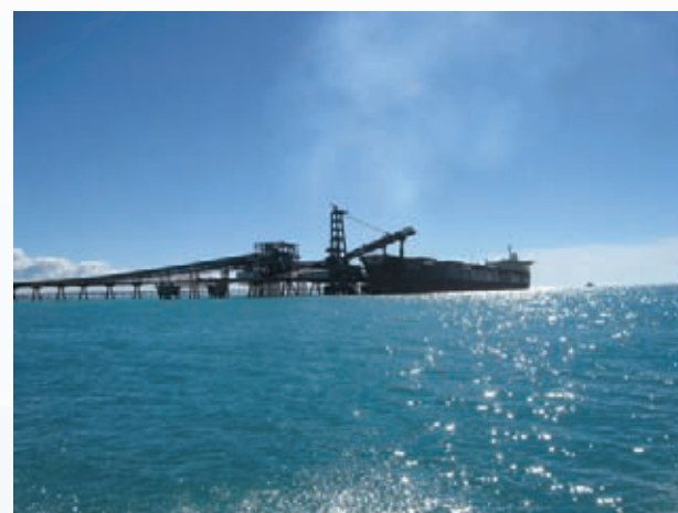
Coal carrier loading at the Port of Hay Point
