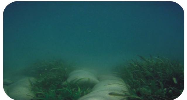
Prop scar restoration in Thalassia meadow using sediment tubes (Seagrass Recovery technology that is being used in Restore a Scar).
