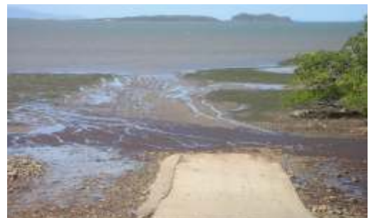
Boat ramp at St Helen's beach. The ramp extends another 300 to 400m at low tide, and is presumably degrading the meadow. Note that the grass on the southern side is much greener, while the prevailing SE wind/current is depositing the mud northwards.
