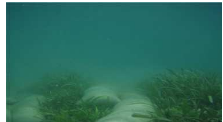
Sediment Tubes installed in propeller scars
