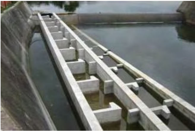
Example of a vertical slot fishway. Photo: Maunsell
